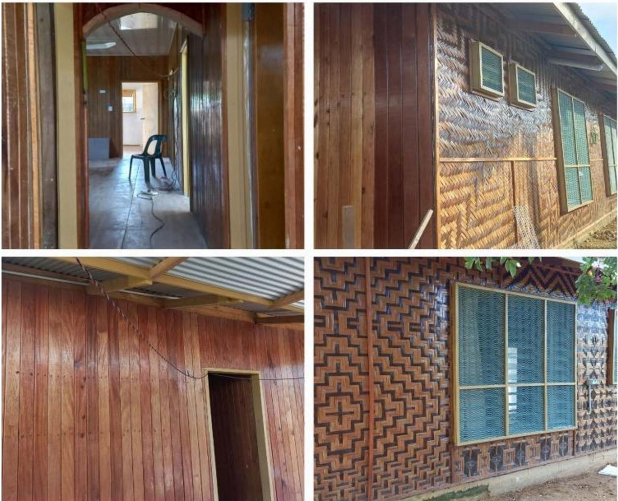
Photos of building and setting up the WCDF.
