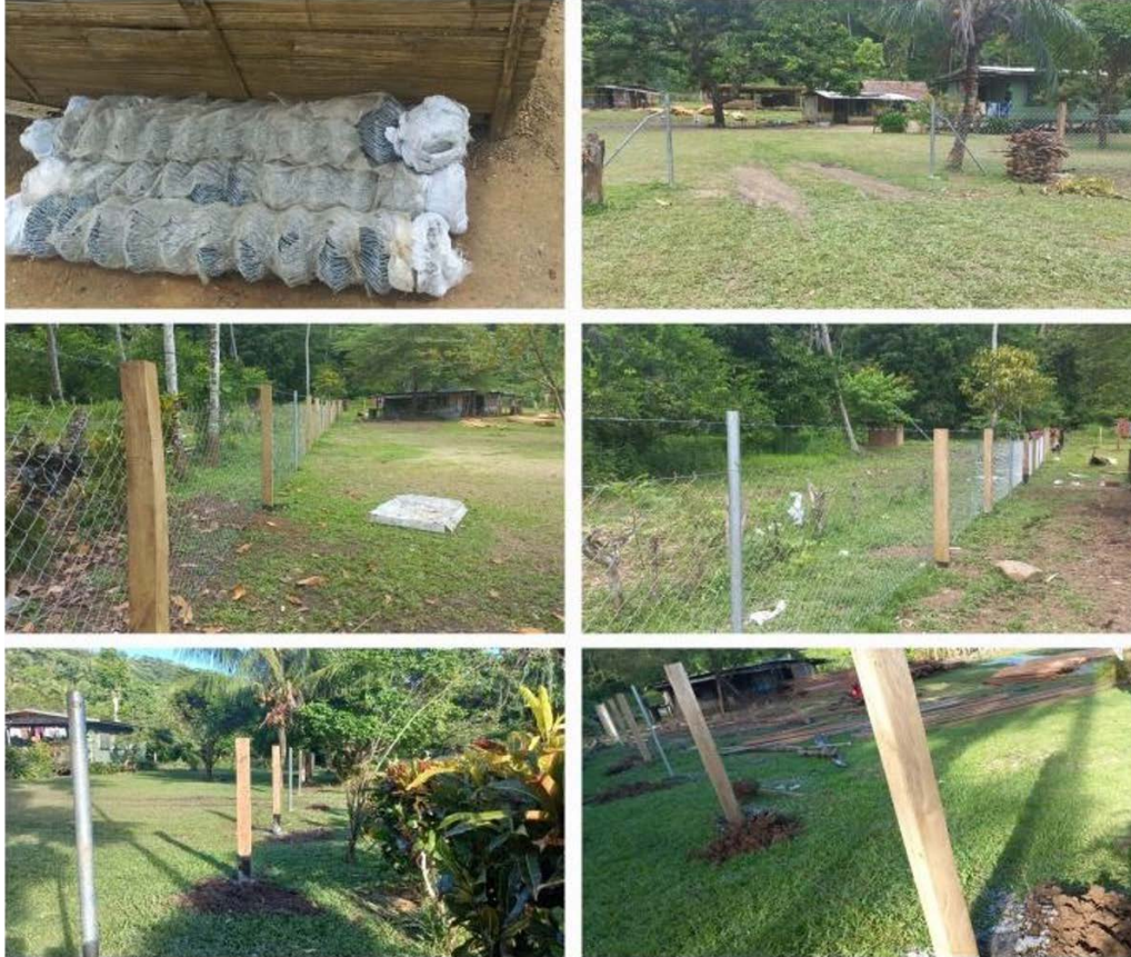
Photos of fencing.
